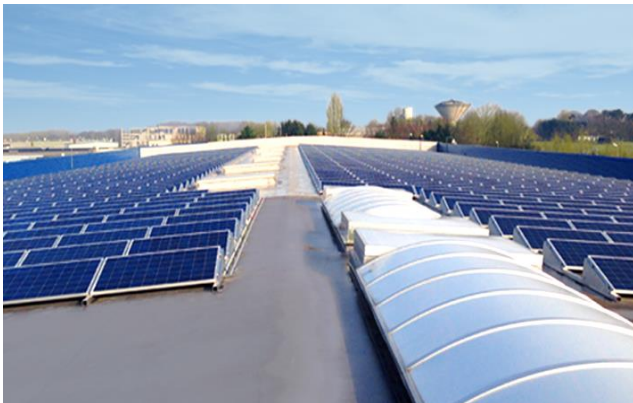
Roof of the STEF Transport Saintes site
