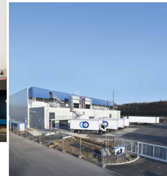
Kölliken under construction
